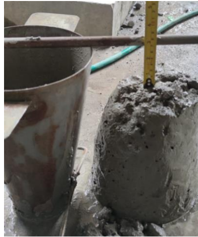
Figure 4. Slump testing on concrete mix
