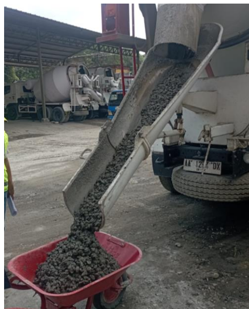
Figure 3. Results of mixing concrete with a mixer truck
