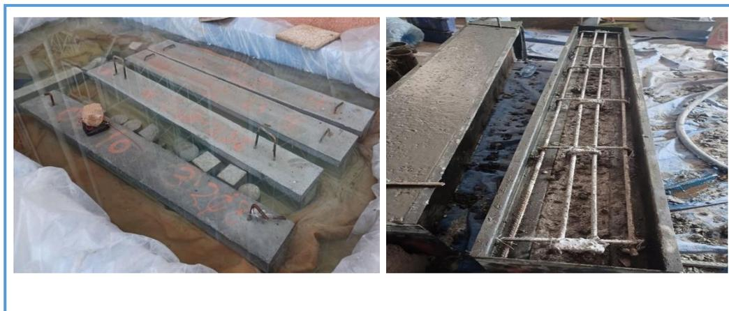
**Figure 4.** beams casting and curing.
