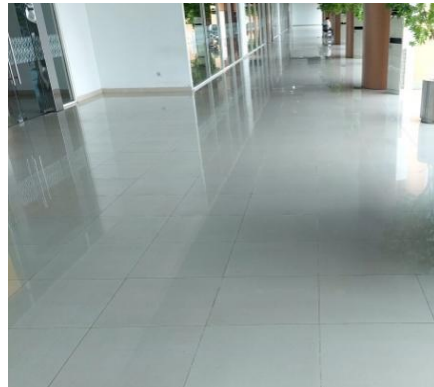
Figure 4. Floor Corridor Gate 3
