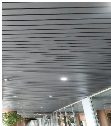
Figure 3. Roof Coridor Gate 3
