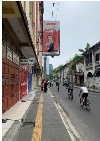
Figure 7. Abandoned and Poorly Maintained Buildings
