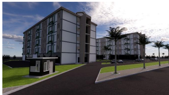
Figure 30. Site Entrance View. (Source: Personal Documentation, 2025)
