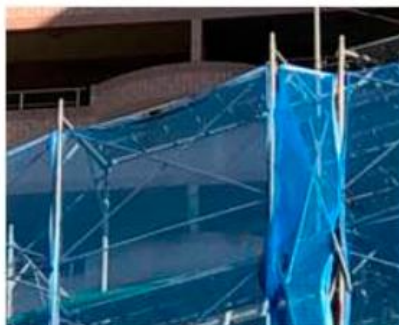
Figure 1. Scaffolding equipped with safety net
