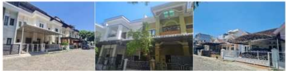
Figure 2. Three Sample Houses Used in the Case Study.
