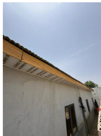
Figure 4. Residential building in Katsina metropolis showing corrugated metal roofing with no insulation and minimal roof overhang a key contributor to indoor heat gain
