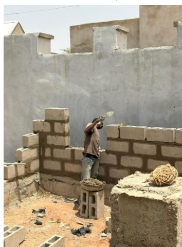
Figure 7. Mason laying mortar on thin sandcrete block wall, demonstrating the shallow wall thickness typical of contemporary residential construction in Katsina — a key factor in poor thermal performance
