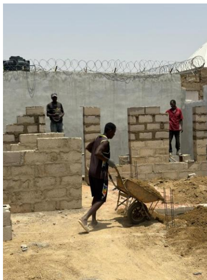
Figure 6. Builders laying sandcrete blocks at an active residential construction site in Katsina metropolis, illustrating the dominance of cement block construction
