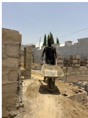
Figure 3. Field data collection at an active residential construction site in Katsina metropolis showing sandcrete block construction in progress
